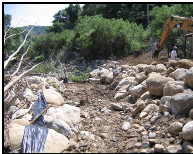
(left) Building riprap. (right) Building riprap.
