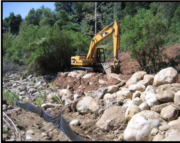
(left) Building rip-rap. (right) Filling rip-rap with soil to facilitate re-vegetation.
