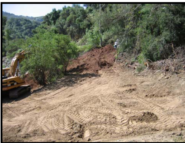
Introduced material used to bring site to grade.
