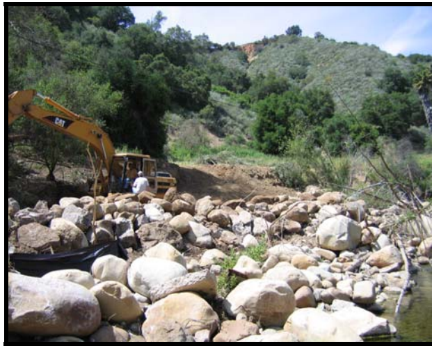
(left) Before: existing boulders onsite. (right) After: boulders removed to use for riprap.
