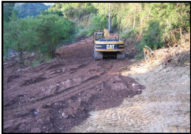
Spreading introduced material to level site.
