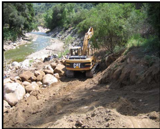
(left) Removing vegetation. (right) Clearing work area of vegetation
